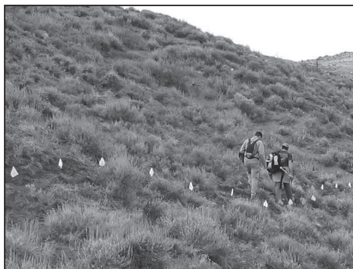
Figure 6—Pin flags mark the exact location of the trail tread and give you a good feel for the flow of the trail.
